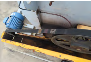
Installing a high-efficiency power transmission system for exhaust fans
